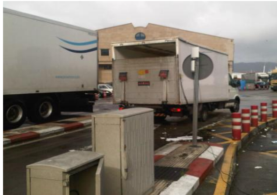
Fig.3: Implemented RSU for trucks (Pole and white antennas)
